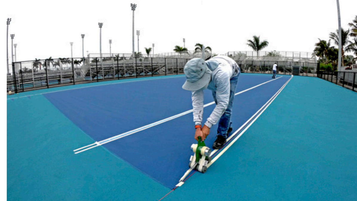
Taping in preparation for line paint
