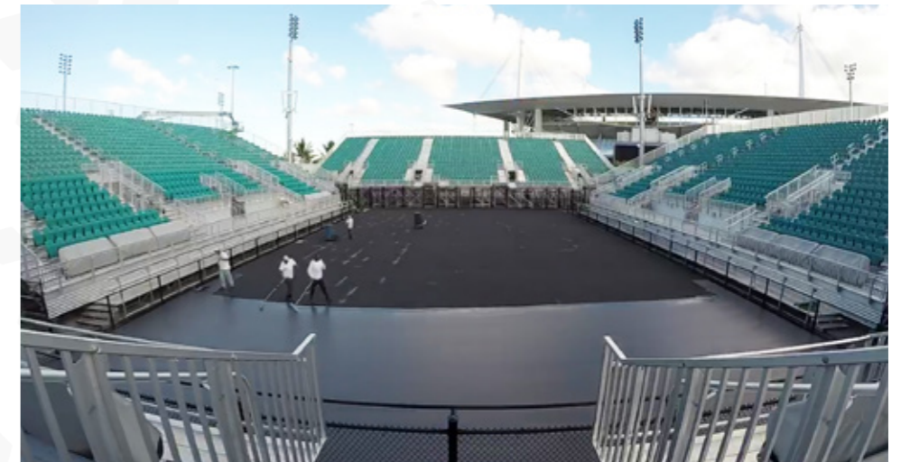
Applying the Laykold Resurfacer
